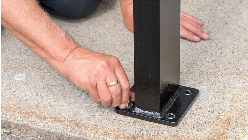
**10** Bolt the bike rack to the anchors with the supplied bolts and metal washers.
