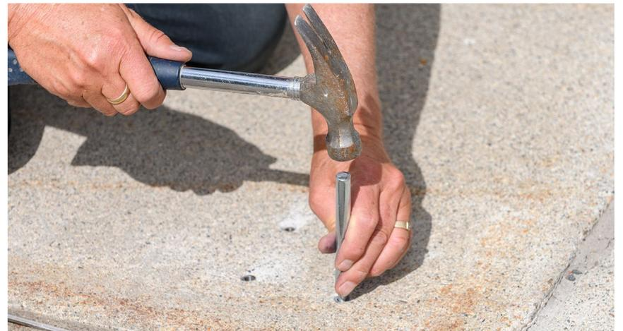
**9** Position the bike rack on the concrete pad by lifting it in place. Line up the holes and ensure the anchors remain free of any debris. Use shims as needed to ensure the bike rack is exactly vertical.
