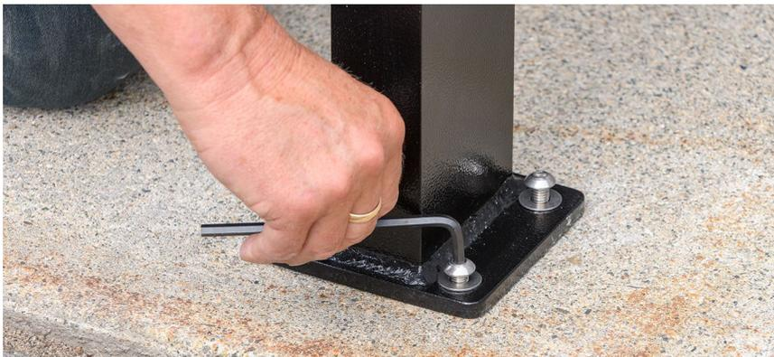
**11** Optional. For theft resistance, fill in the bolt heads with silicone and paint the tops of the fasteners with a paint pen to match the colour of the bike rack.
