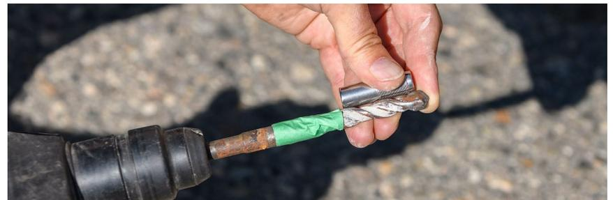
**5** Drill all holes to the depth indicated by the tape or marker applied to the drill in step 4. Holes must be vertical to properly anchor the bike rack.
